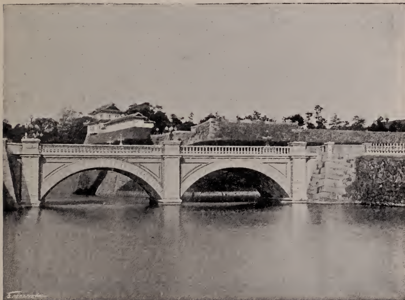
APPROACH TO THE PALACE
